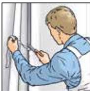
**6.** Trim off excess wallpaper at the corners and edges and butt joint the next length.
