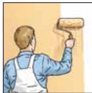
**7.** When dry, apply one or two coats of high-quality emulsion paint (DIN EN 13300-compliant).
