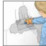
6. Fill the joints between the panels with ERFURT-KlimaTec SR 6 system adhesive.
