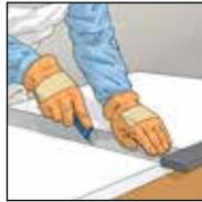
2. Use a Stanley knife to scarify the insulating wedge and break at the edge or cut with a saw.
