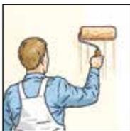
7. Prime the insulating wedge with paste.
