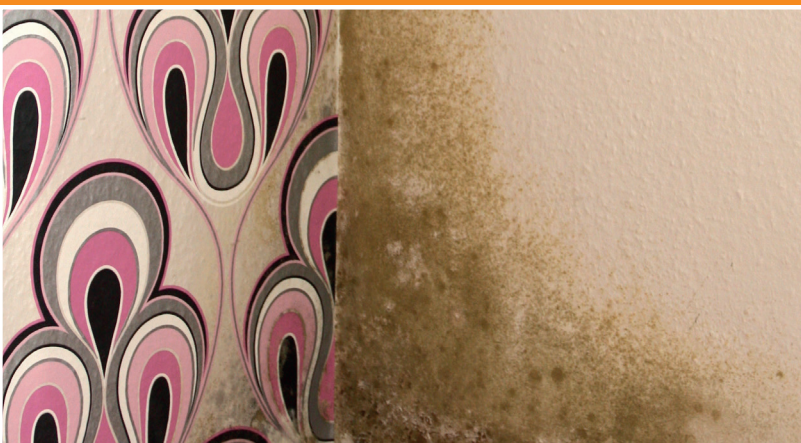
Schimmelbefall | Mould growth
